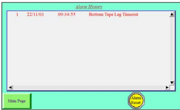
Figure 51: HMI Alarm History Screen
